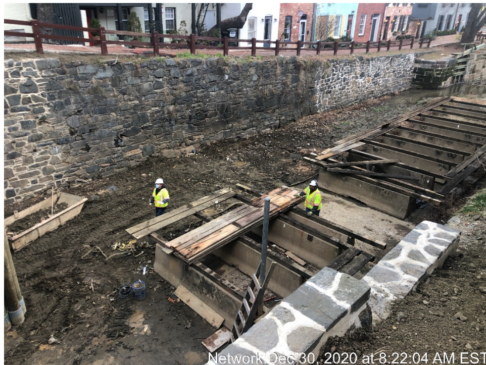
Restoring the Concrete Barriers at the Boat Section
