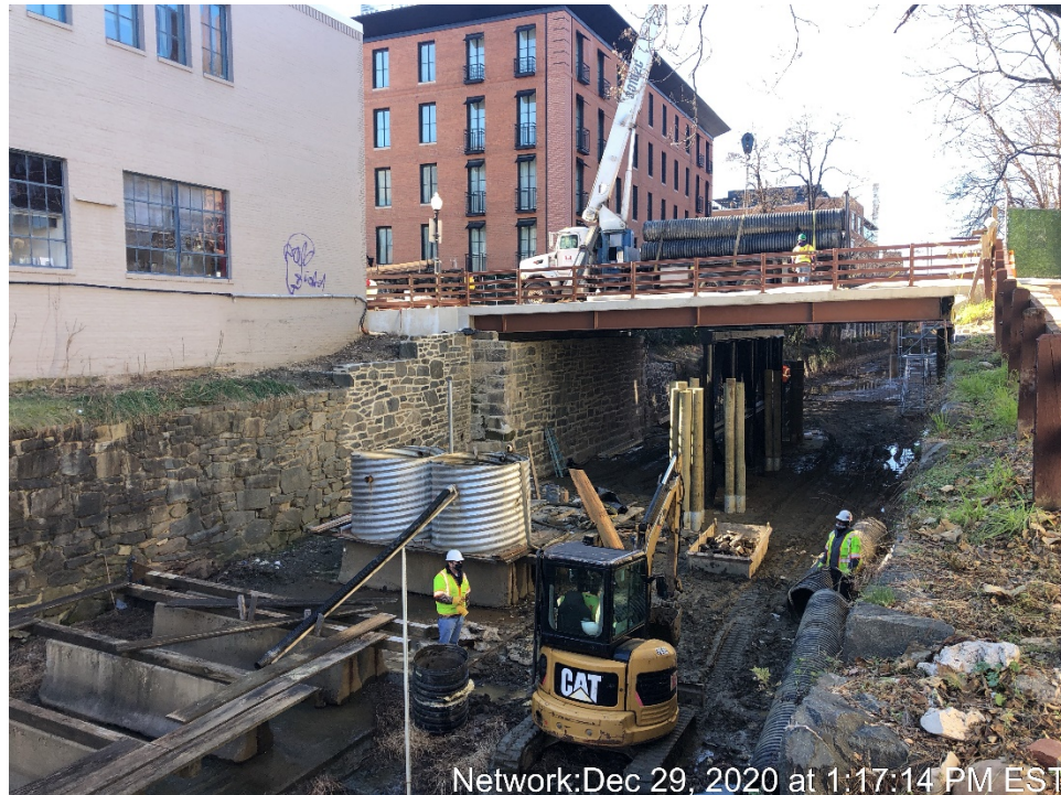
Removal of the 24-inch Conveyance Pipe
