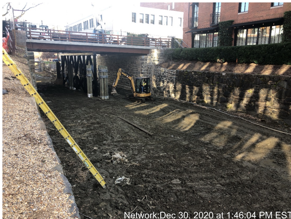
Grading at the Bottom of the Canal
