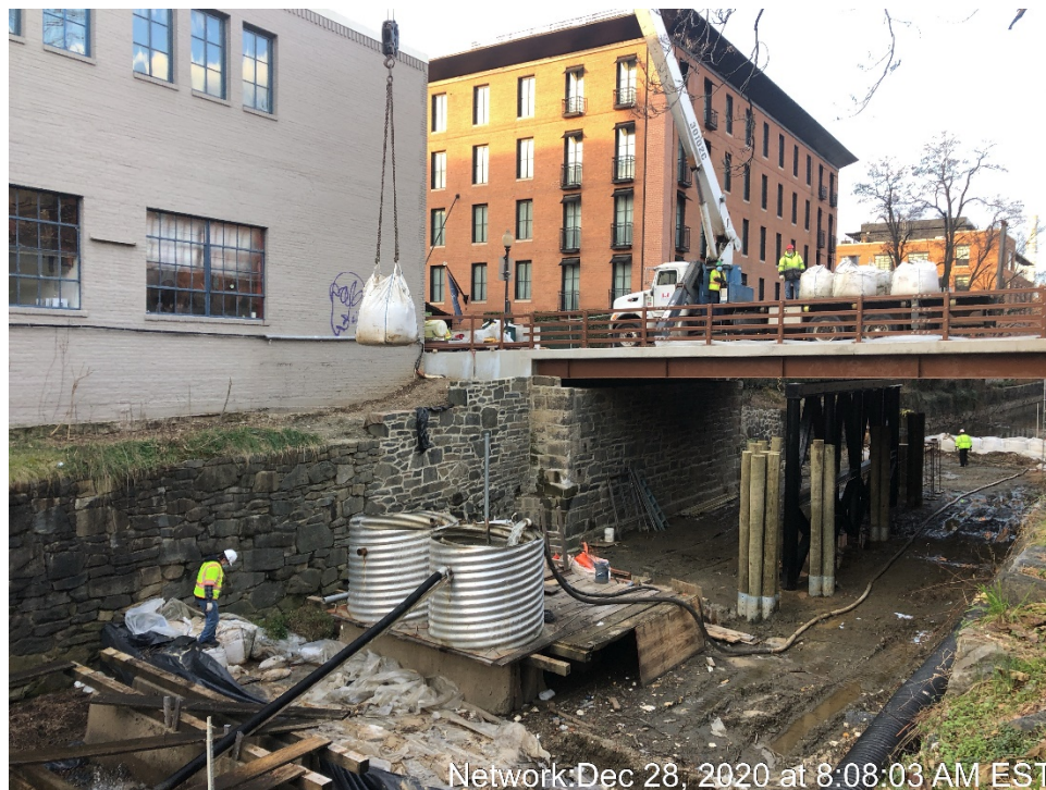
Removal of Downstream Cofferdam
