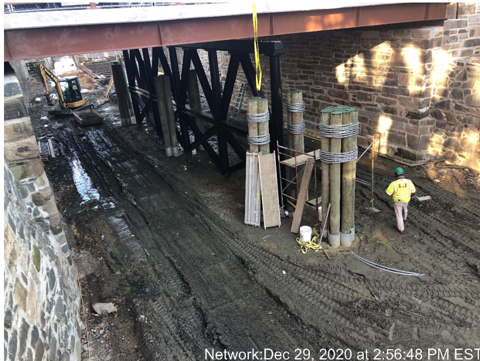
Grading the Canal Bed
