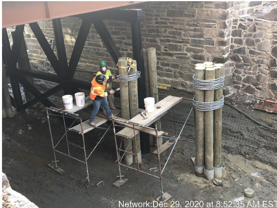
Installation of Wire Rope Around the Dolphins
