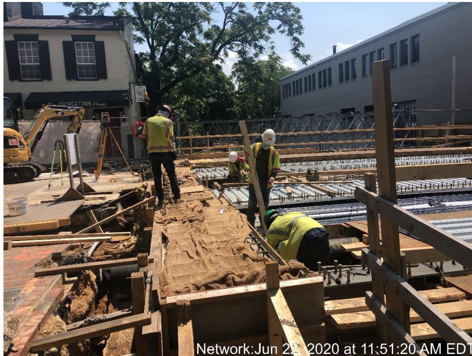
Formwork Removal at the North Abutment Back Wall
