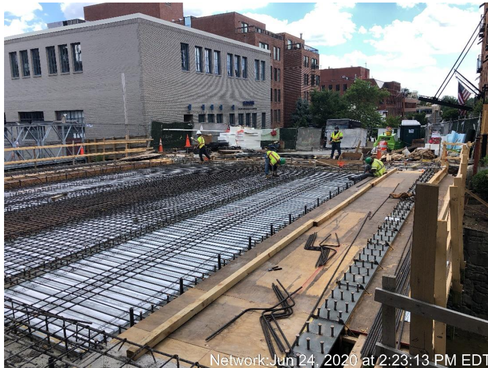
Placement of Reinforcing Steel for the Bridge Deck
