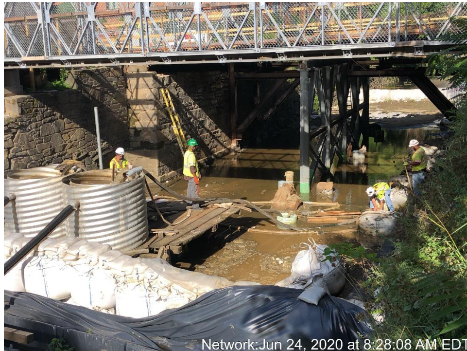
Dewatering the Flooded Work Zone
