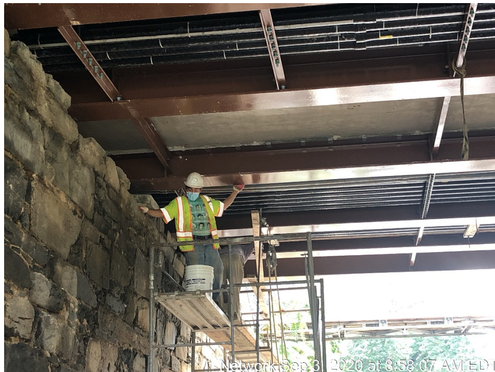
Repointing at North Canal Wall
