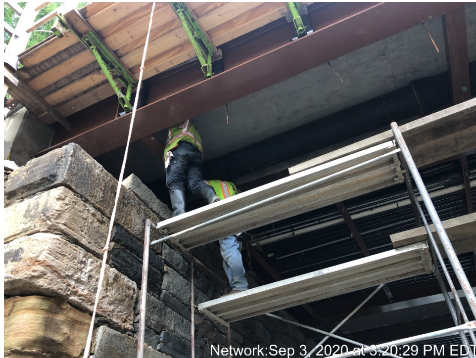
Repointing at North Canal Wall
