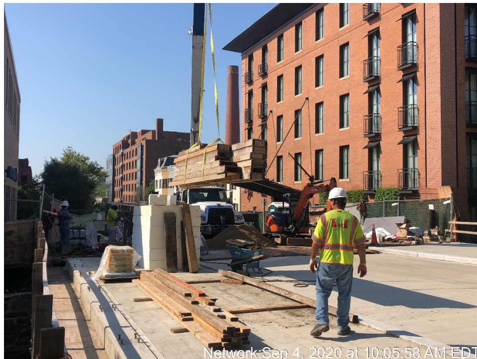
Removal of the Formwork Debris
