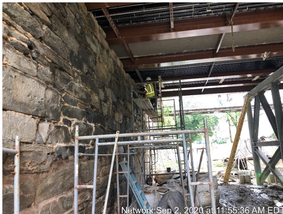
Repointing at North Canal Wall
