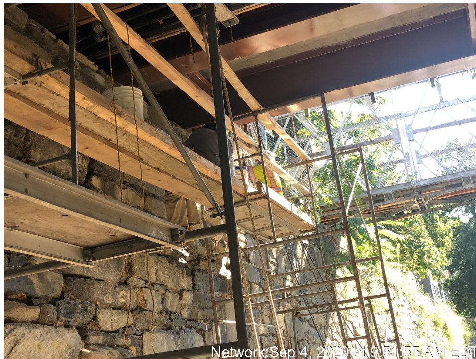
Repointing at North Canal Wall
