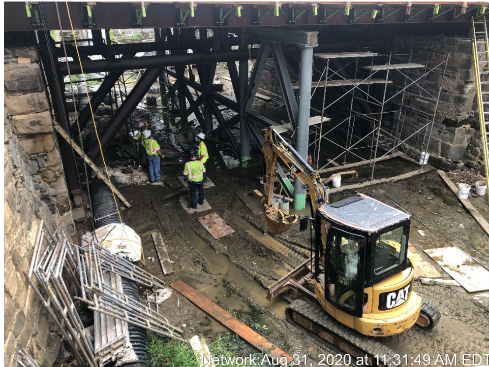
Network: Aug 31, 2020 at 11:31:49 AM EDT Removal of Temporary Utility Support
