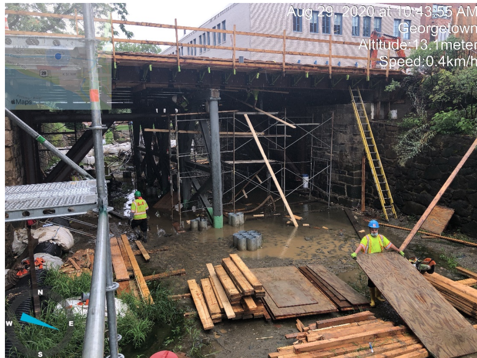
Removal of Temporary Utility Support and Formwork
