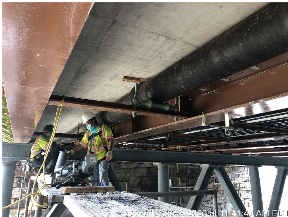
Installation of Diaphragm Connection under 12-inch Water Main
