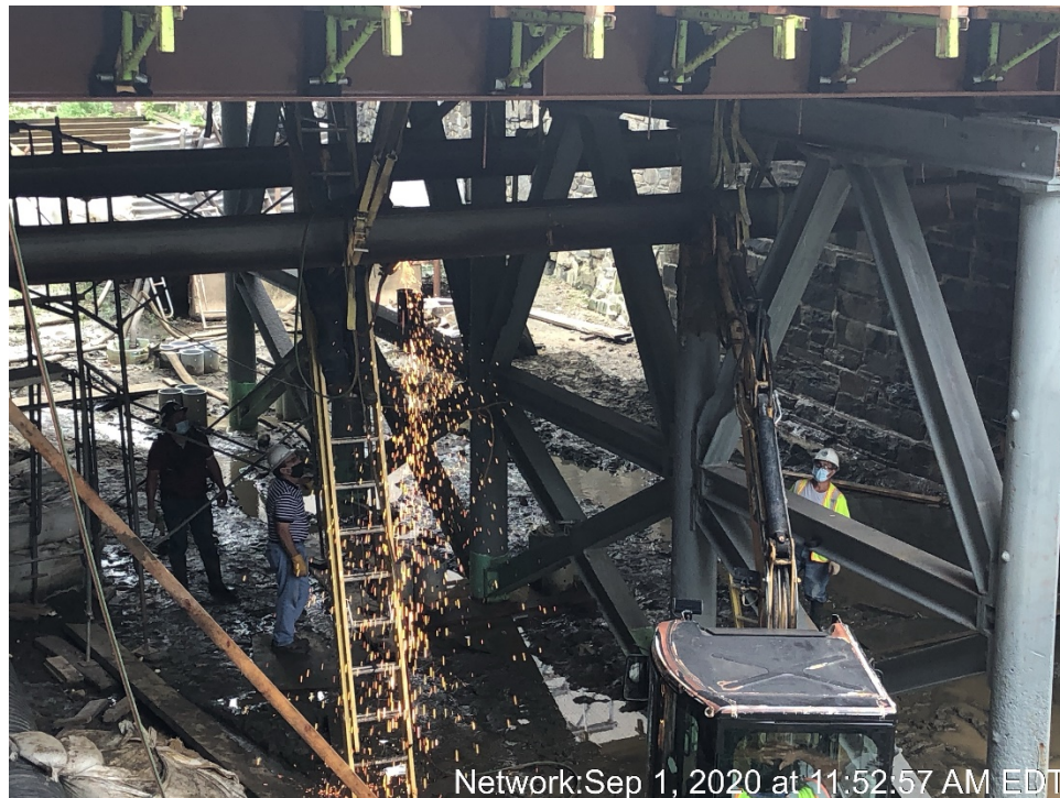
Network: Aug 31, 2020 at 11:31:49 AM EDT Removal of Temporary Utility Support
