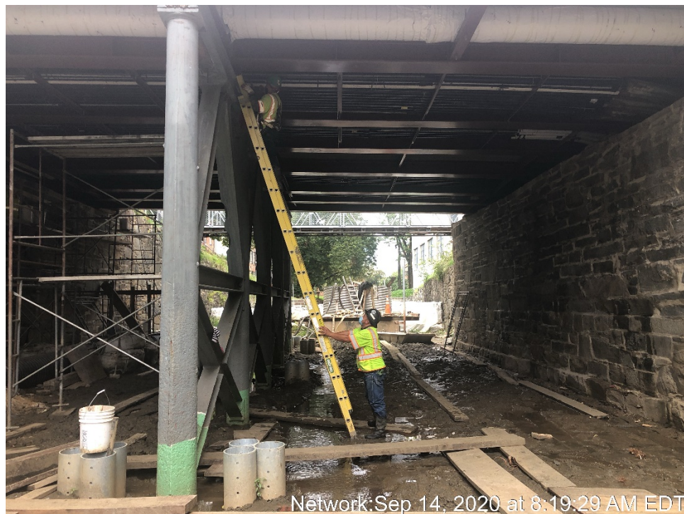
Cleaning and Paint Touch Up for Beams Beneath the Bridge
