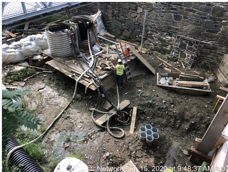
Network: Sep 15, 2020 at 9:46:57 AM EDT Repointing at North Canal Wall
