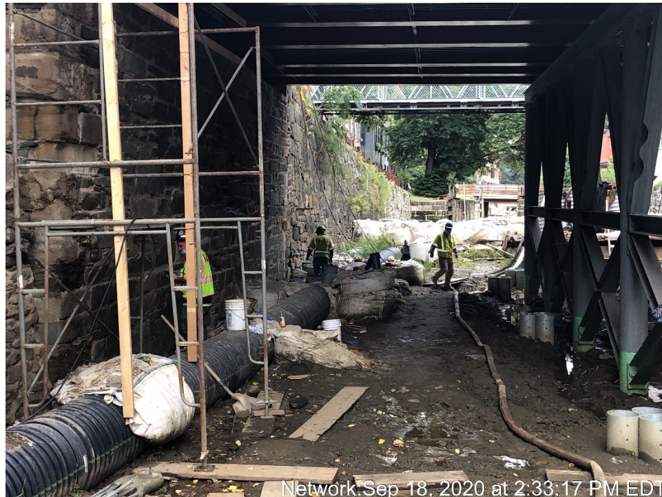
Repointing at North Canal Wall
