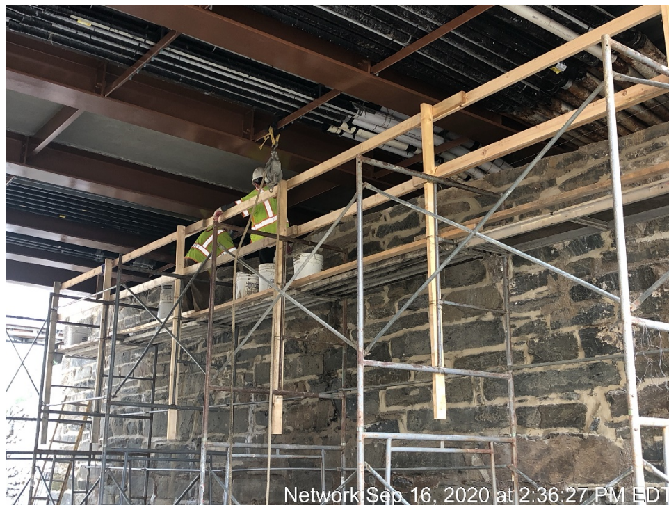
Repointing at South Canal Wall
