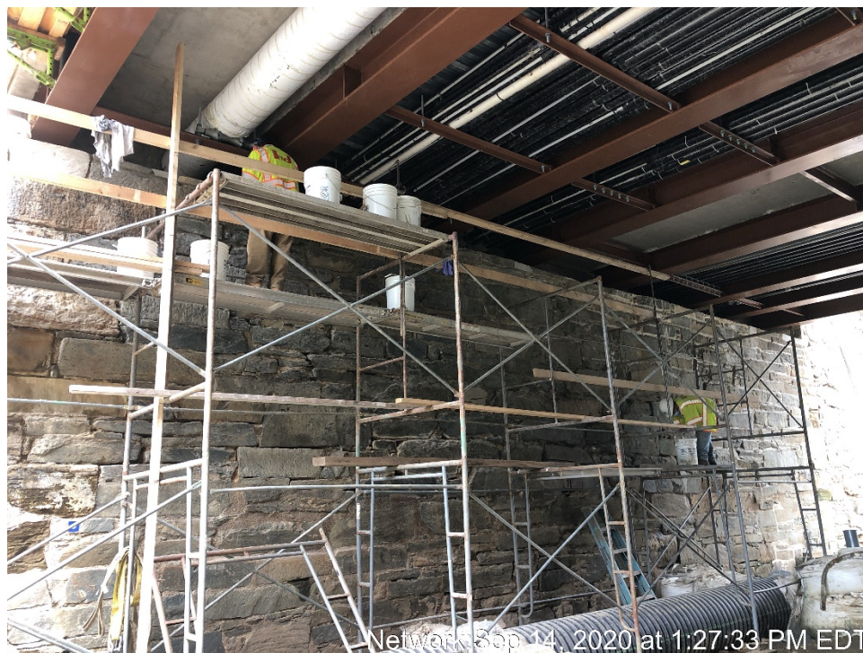
Repointing at North Canal Wall
