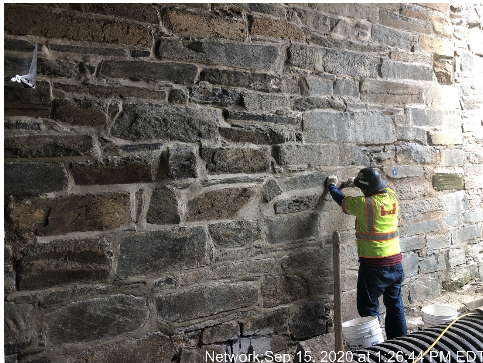
Repointing at North Canal Wall
