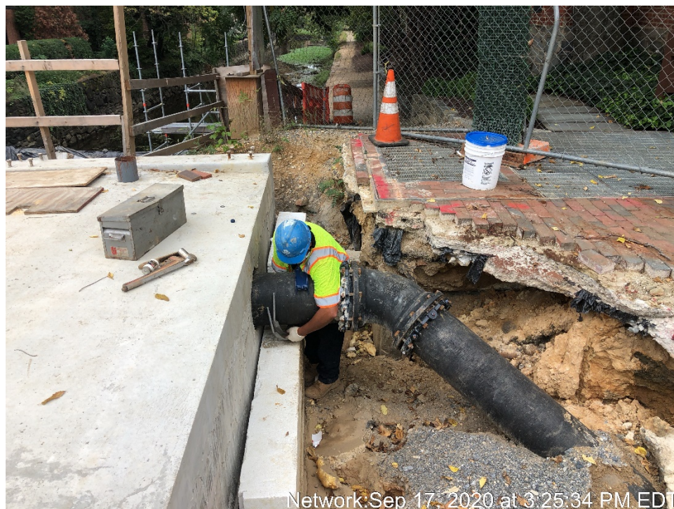
Tie-in for the 12-inch Water Line at the North abutment
