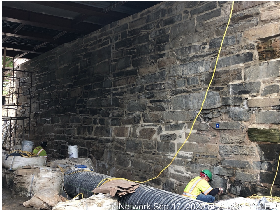
Repointing at North Canal Wall
