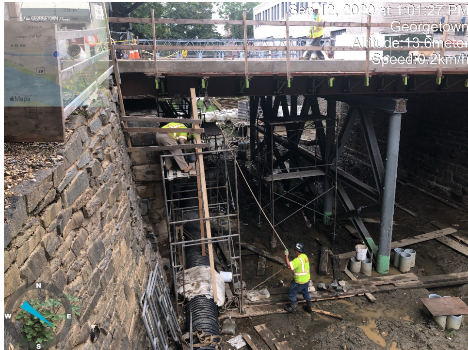
Repointing at the North Canal Wall
