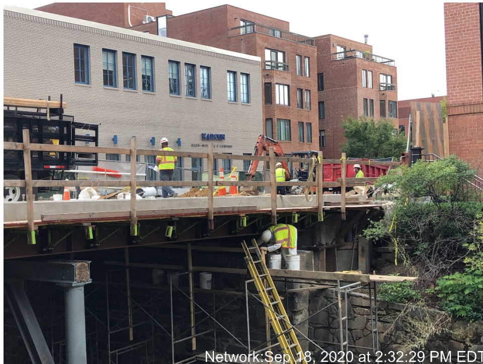
Network: Sep. 18, 2020 at 12:52:20 PM EDT Density Checking for the 12-inch Water Main Backfill at the South Abutment
