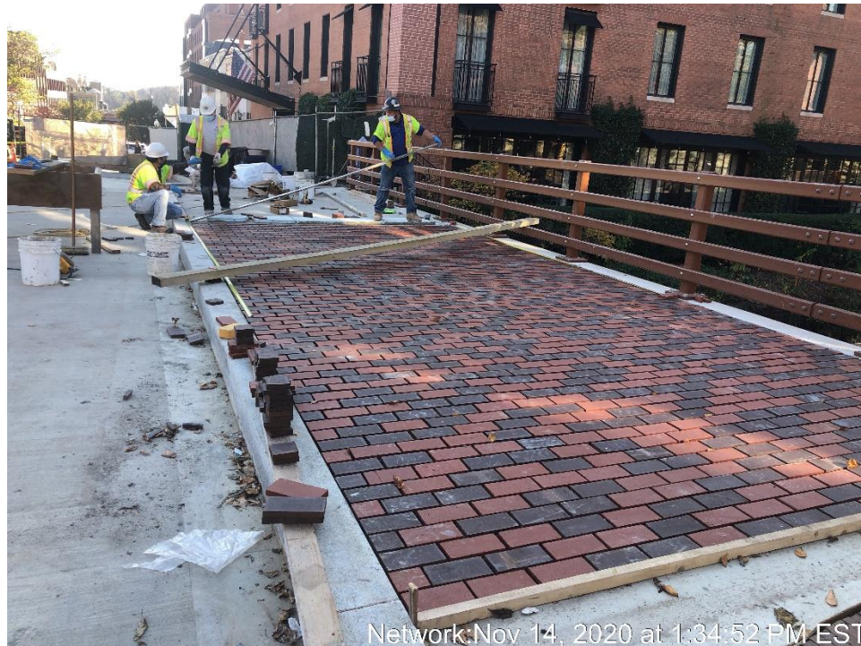
Construction of Brick Sidewalk – West Side of the Bridge
