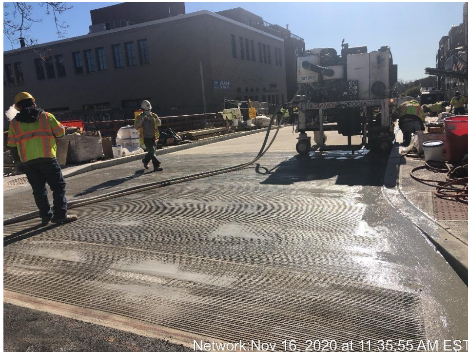
Grooving at the North Approach Slab
