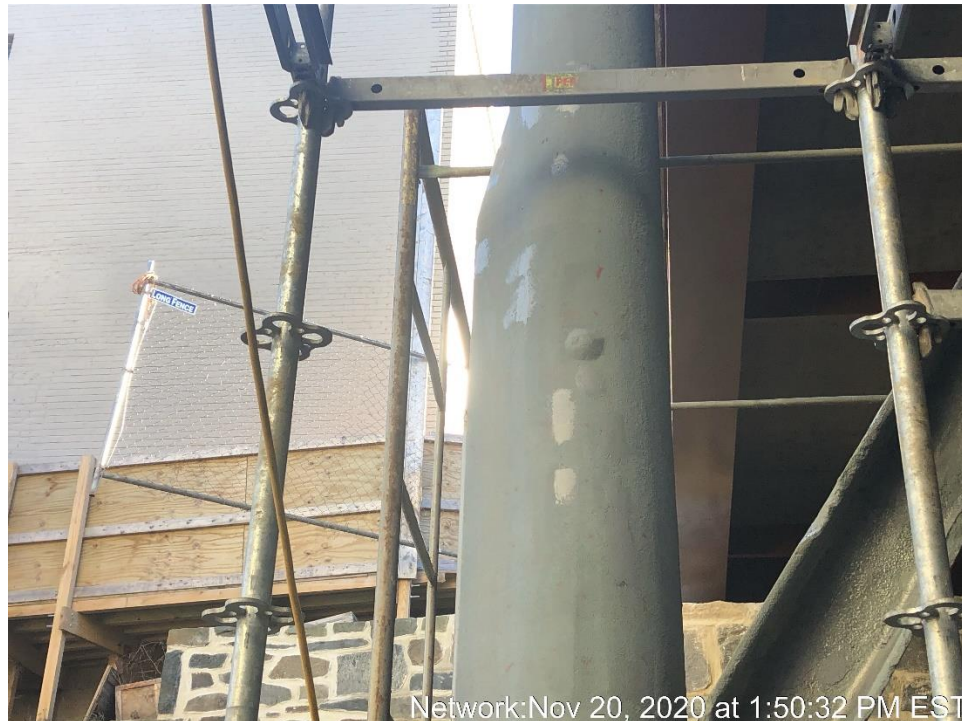
Epoxy Hole Filling at Pier Column
