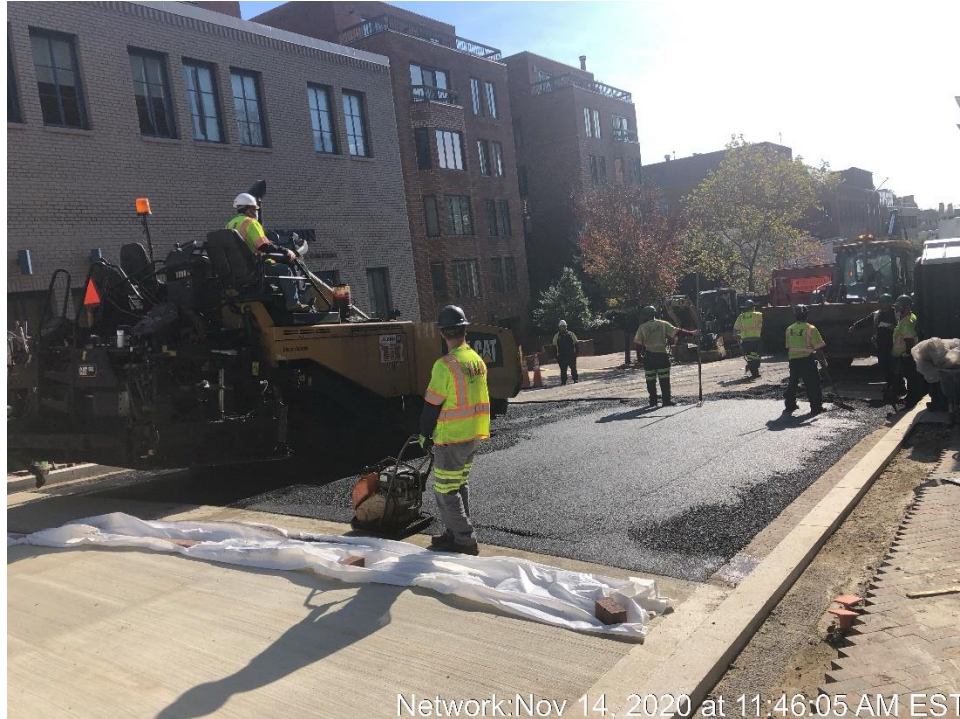
Placement of Asphalt at South Side of the Bridge
