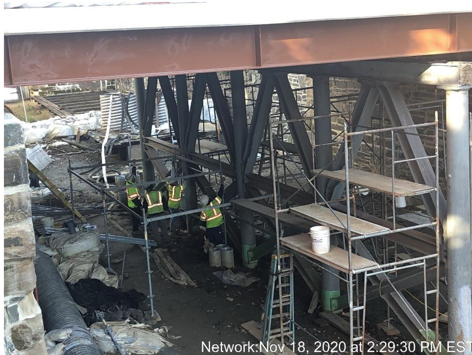
Scaffolding and Containment for Pier Epoxy Repairs
