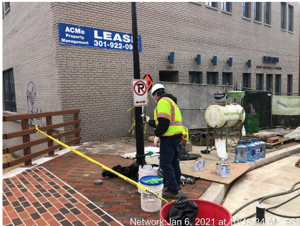
Repainting the Existing Light Pole at the SE Side of the Bridge
