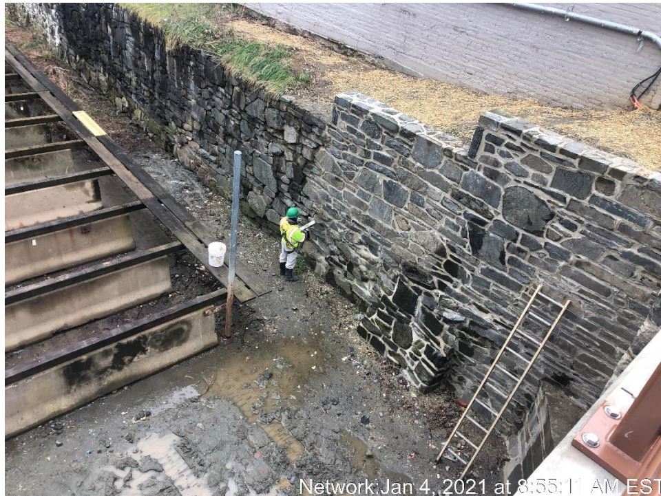
Repointing Stone Cracks at the South Canal Wall
