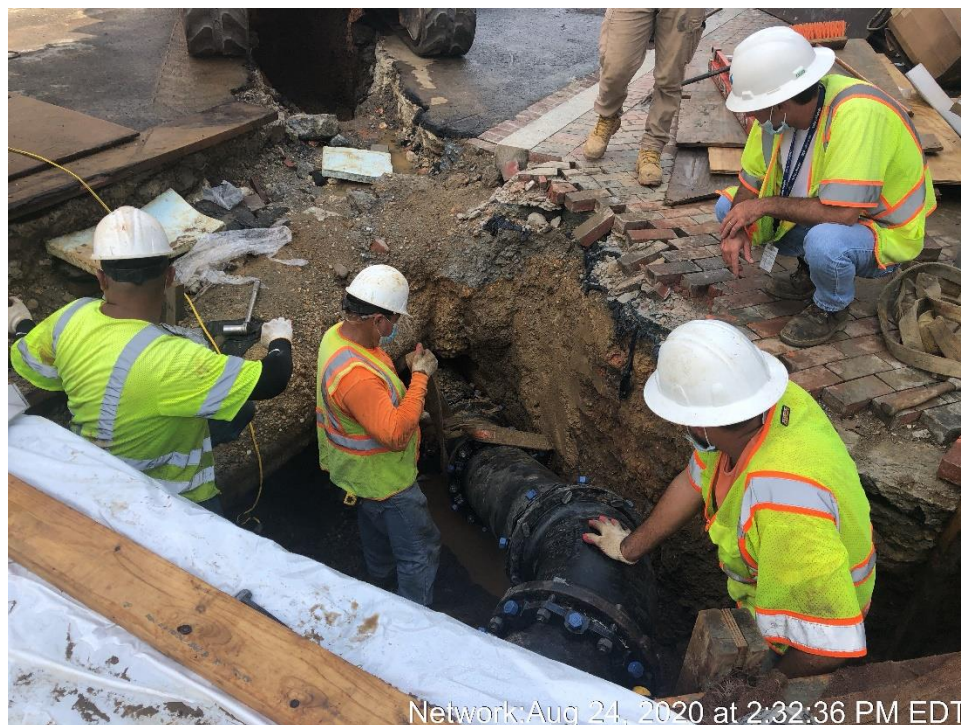
Network: Aug 17, 2020 at 1:01:27 PM EDT Installation of 12-inch Water Main at North Side of the Bridge
