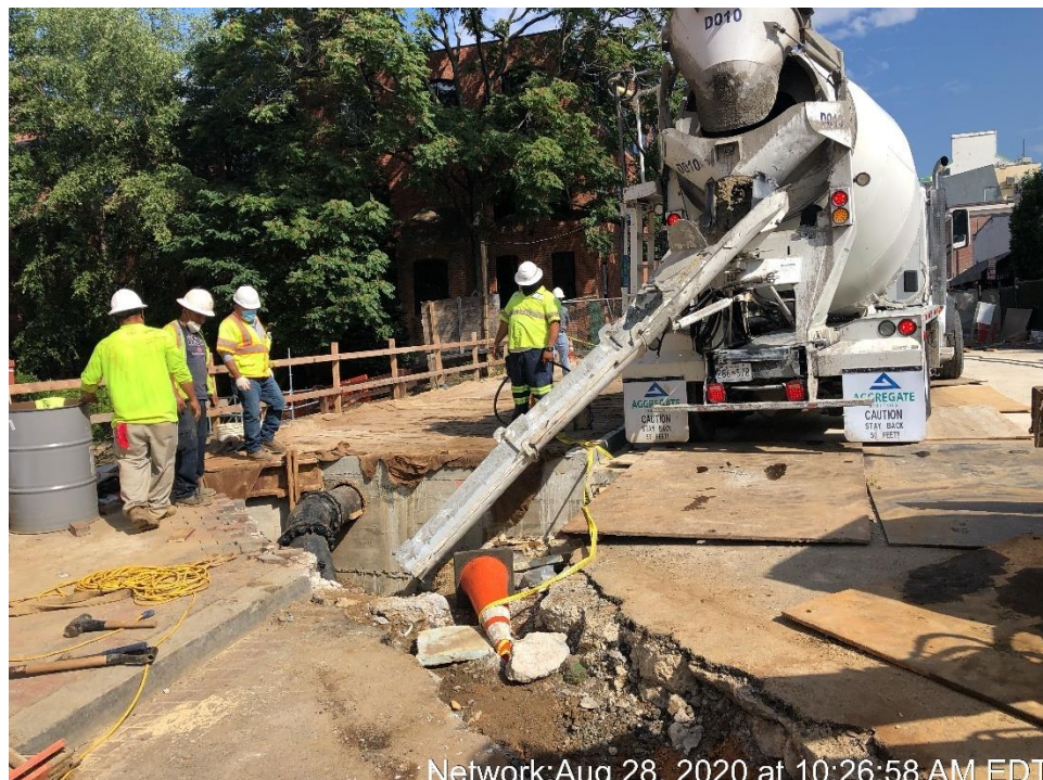
Placement of Flowable Fill Around the Water Main Under Verizon Cables
