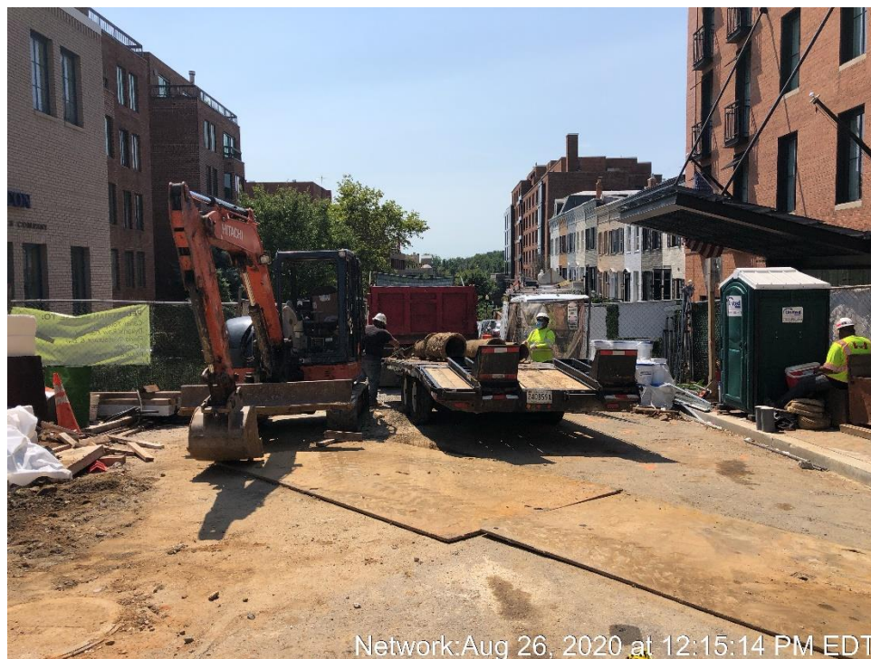
Removal of Water Line Debris
