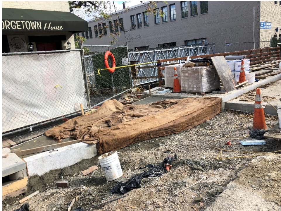
Curing of concrete for ADA-Compliant Ramp at the NE Corner
