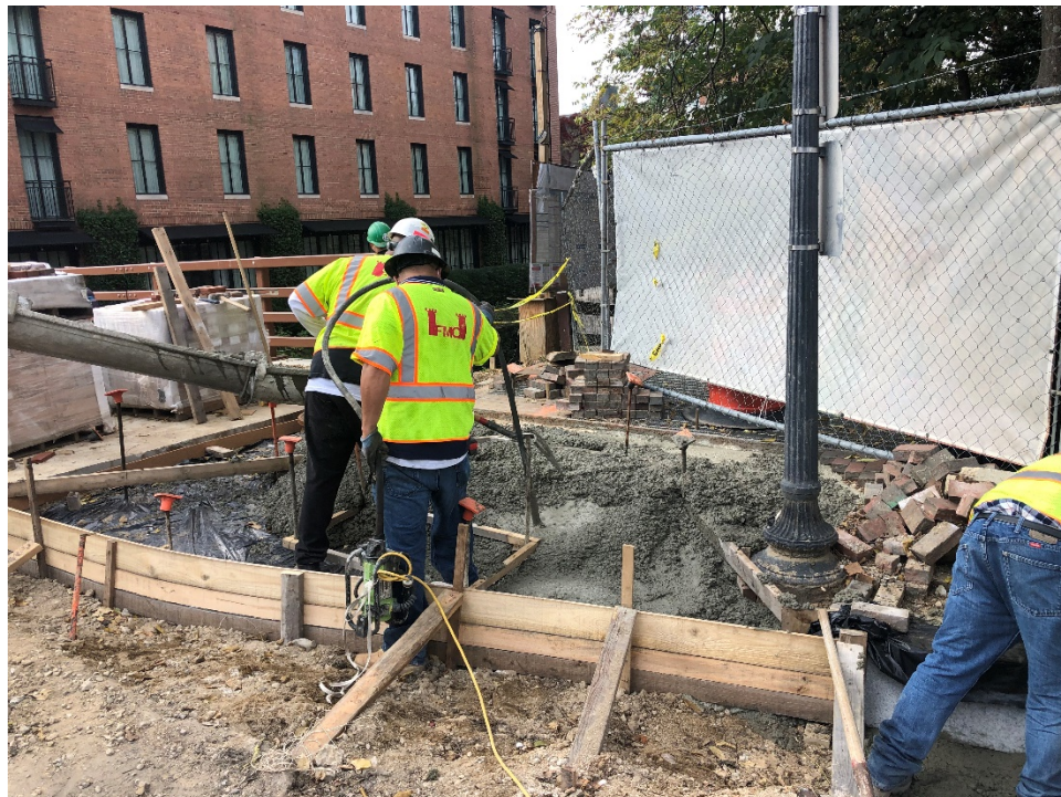
Placement of Concrete for ADA-Compliant Ramp at the NW Corner
