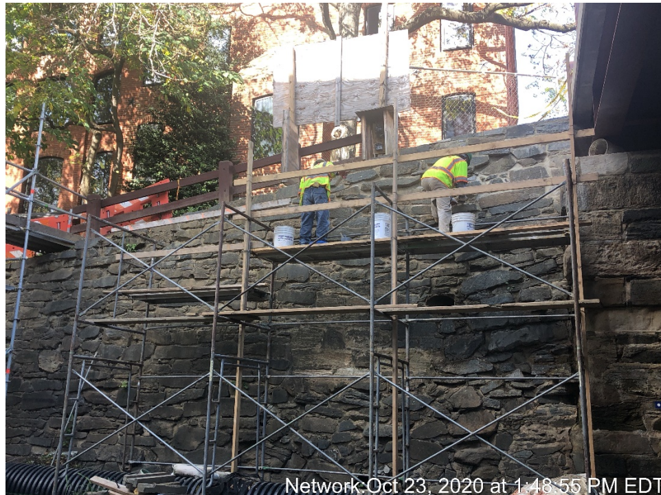
Repointing of Canal North Wall
