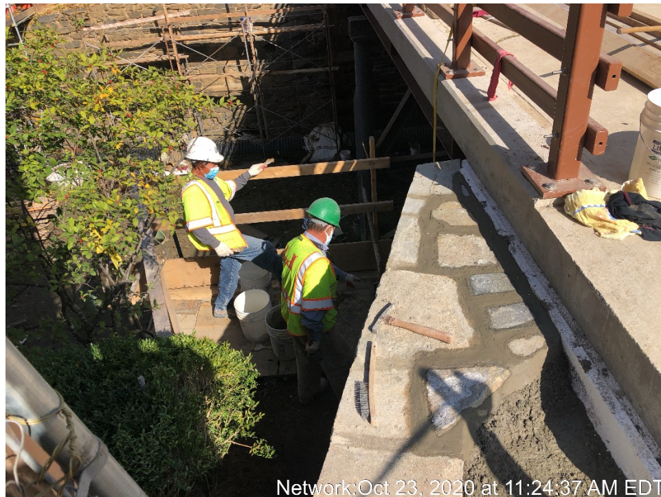
Network: Oct 23, 2020 at 9:55:09 AM EDT Construction of SW Wing Wall
