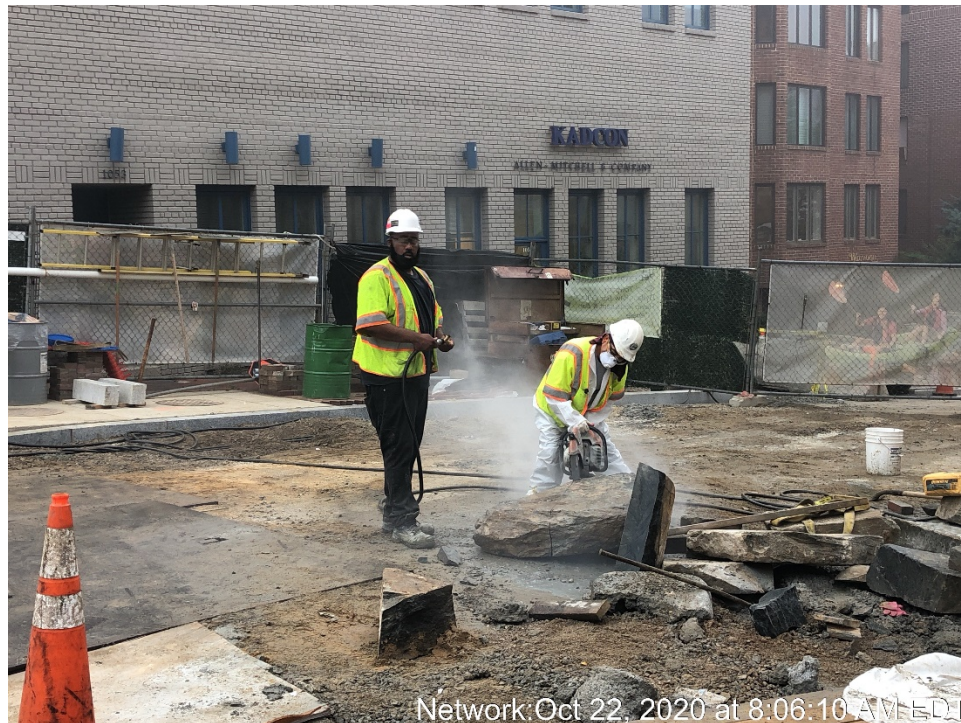
Construction of SW Wing Wall (Stone Cutting)
