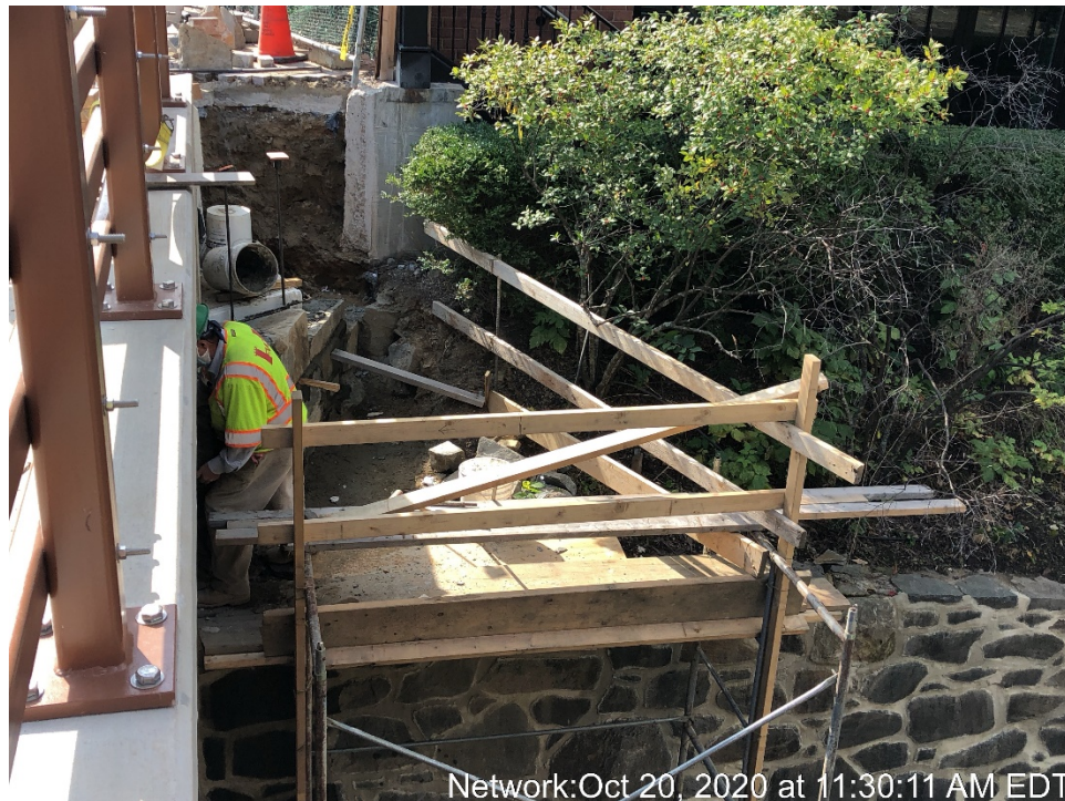
Construction of SW Wing Wall
