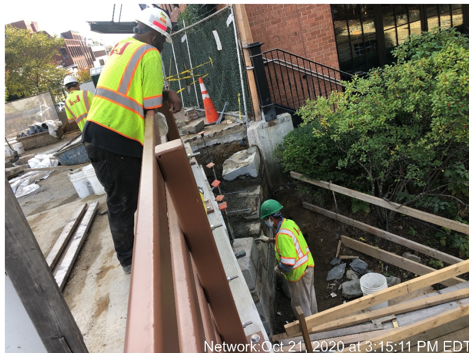
Construction of SW Wing Wall
