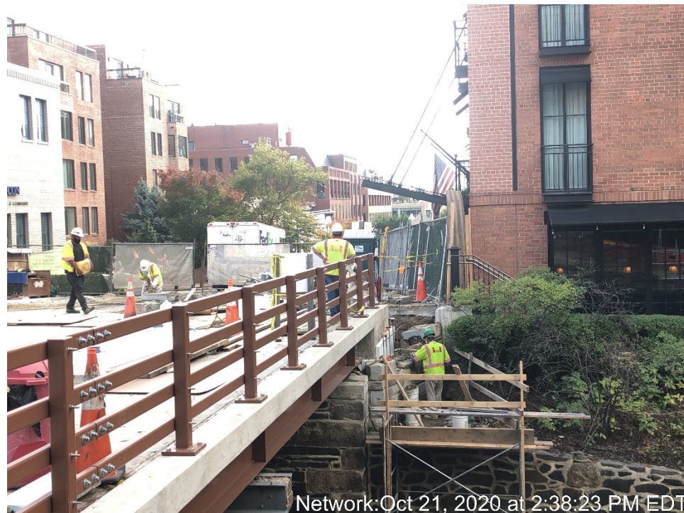
Construction of SW Wing Wall
