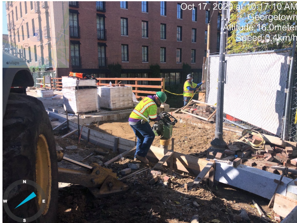
Construction of ADA-Compliant Ramps at NE & NW sides of the Bridge
