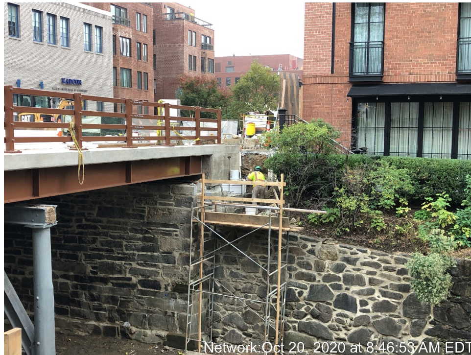
Construction of SW Wing Wall
