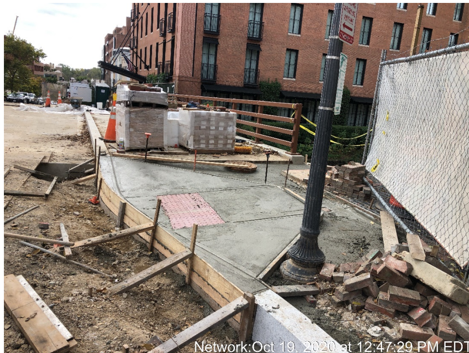
New ADA-Compliant Ramp at the NW Corner
