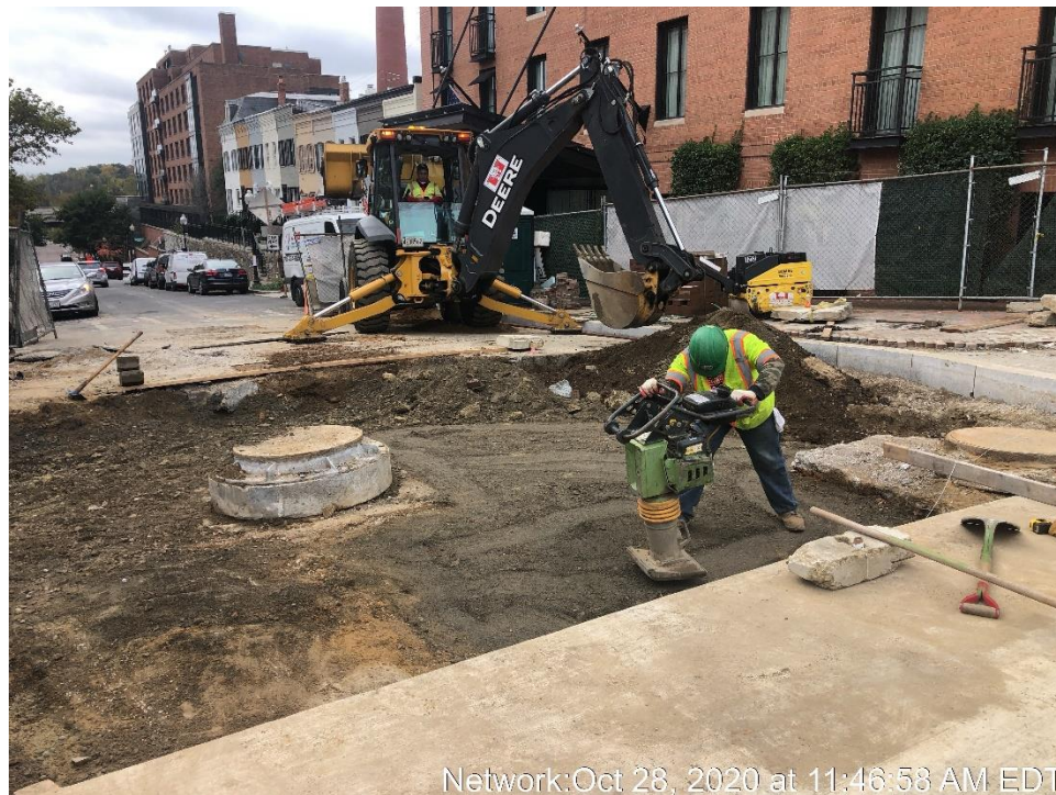
Placement and Compaction of Aggregate for Approach Slab
