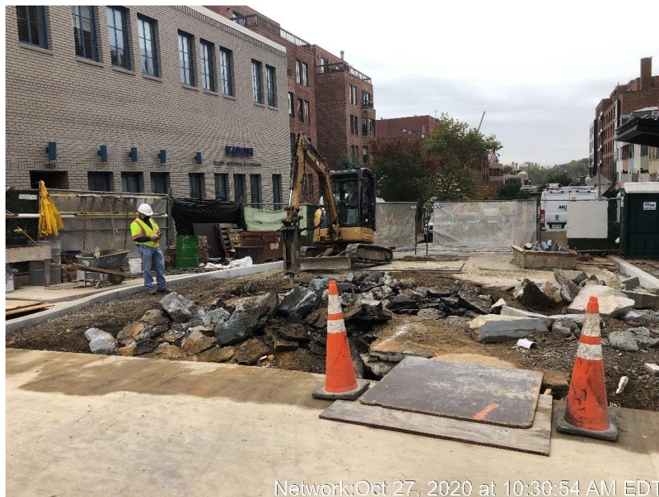
Excavation for the Approach Slab South of the Bridge
