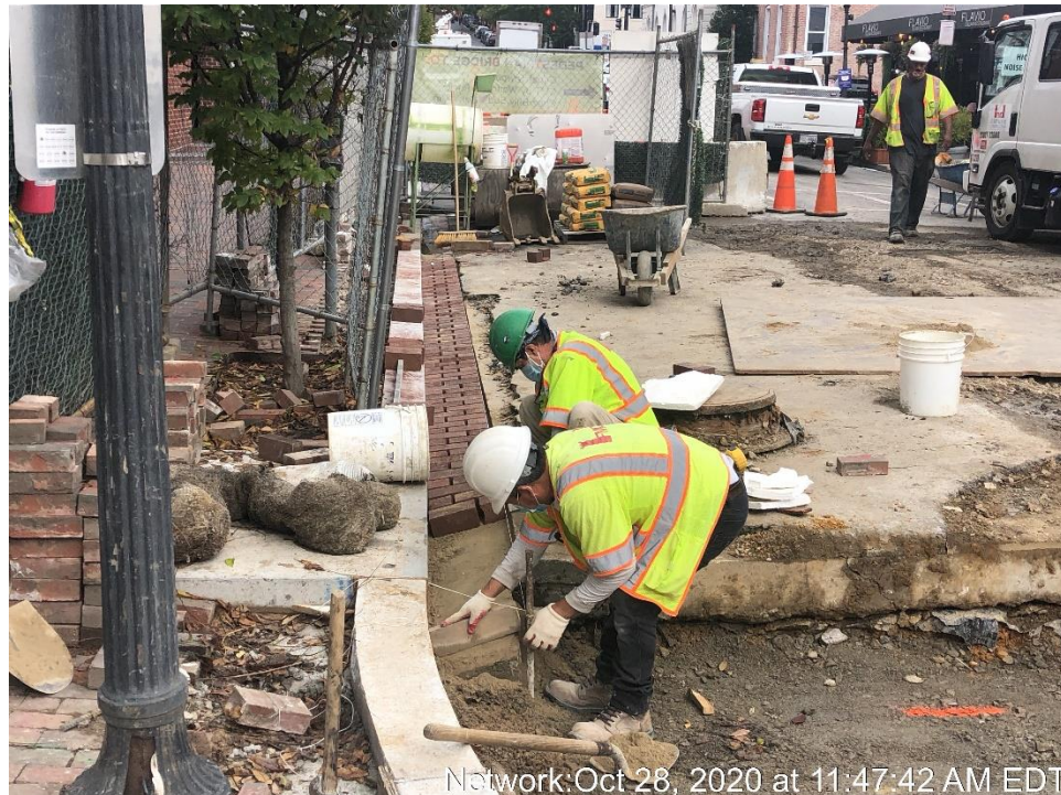
Installation of Brick Gutter
