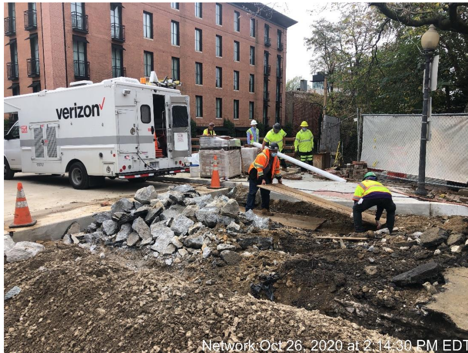
Verizon Encasing Existing Conduit North of the Bridge
