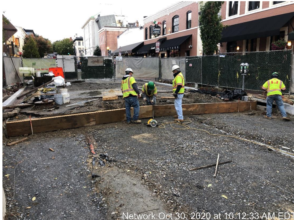
Installation of Formwork for the Approach Slab
