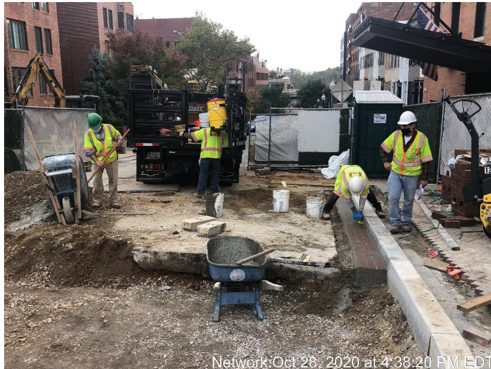
Installation of Brick Gutter at SW Corner
