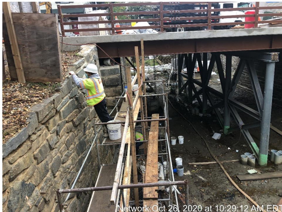
Repointing of Canal North Wall
