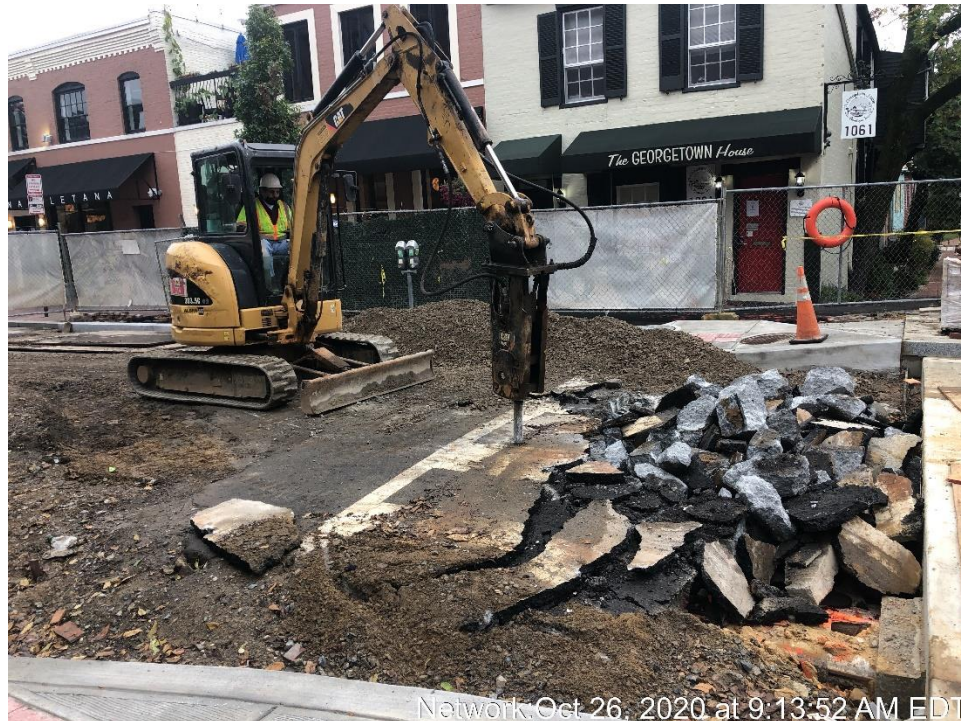
Excavation for the Approach Slab North of the Bridge
