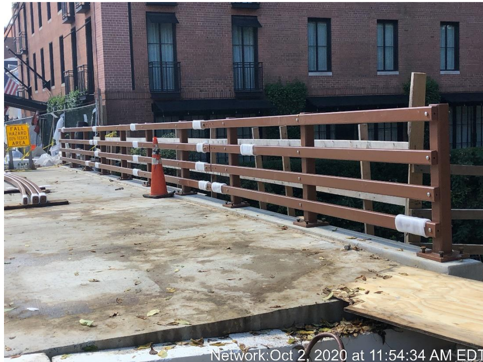
Installation of Railing at the West Side of the Bridge
