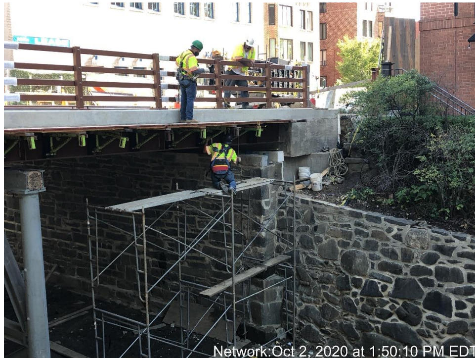
Removal of Overhang and Wood Platform West side of the Bridge
