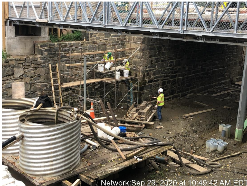
Network: Sep 29, 2020 at 10:03:02 AM EDT Repairing and Repointing at the South Canal Wall
