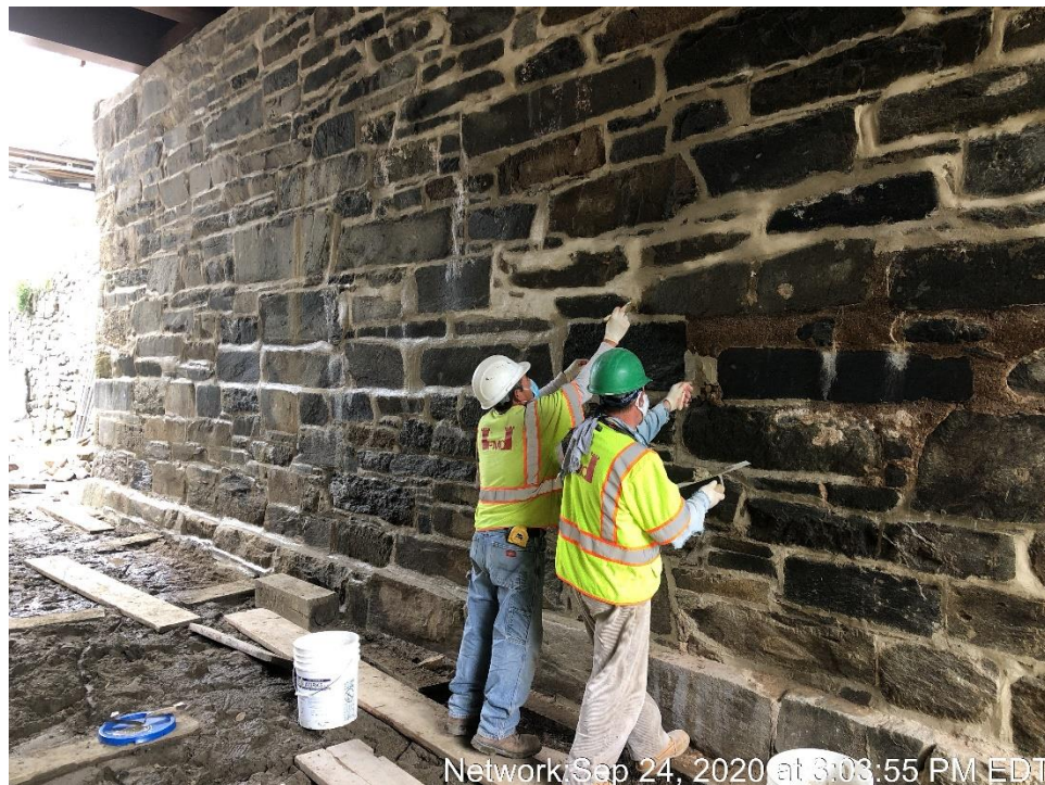
Repairing and Repointing at the South Canal Wall
