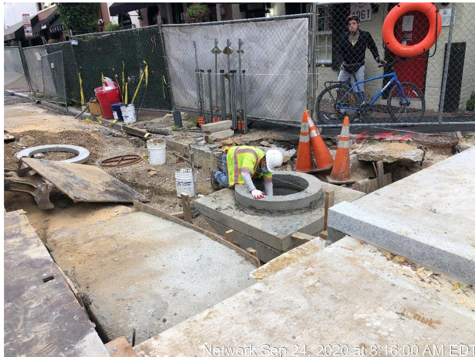
Adjusting Frame and Cover for Pepco Manhole North of the Bridge
