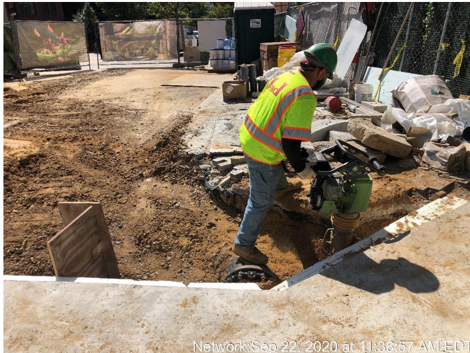
Backfill for the Water Line Trench South of the Bridge
