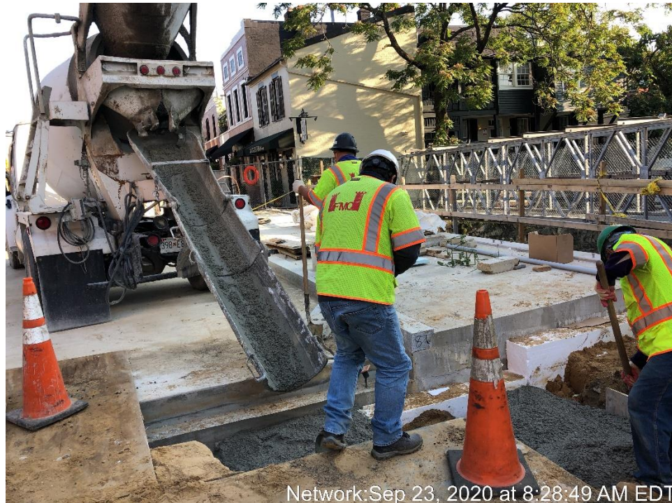
Placement of Flowable Fill Concrete at the South Abutment
