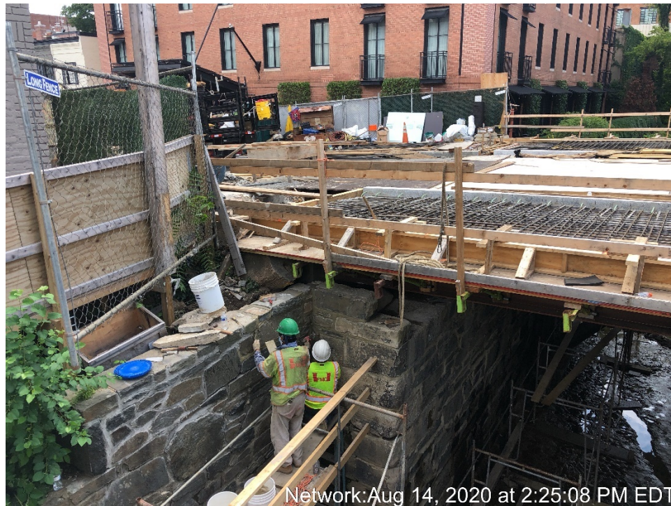
Repointing Canal Wall Stone at the South Abutment
