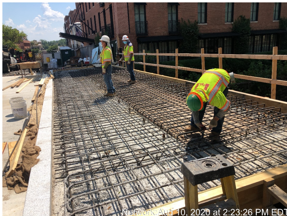
Placement of Reinforcing Steel for Sidewalk
