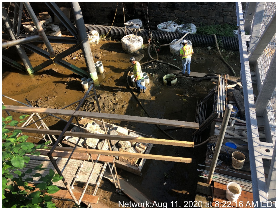
Dewatering the Work Zone
