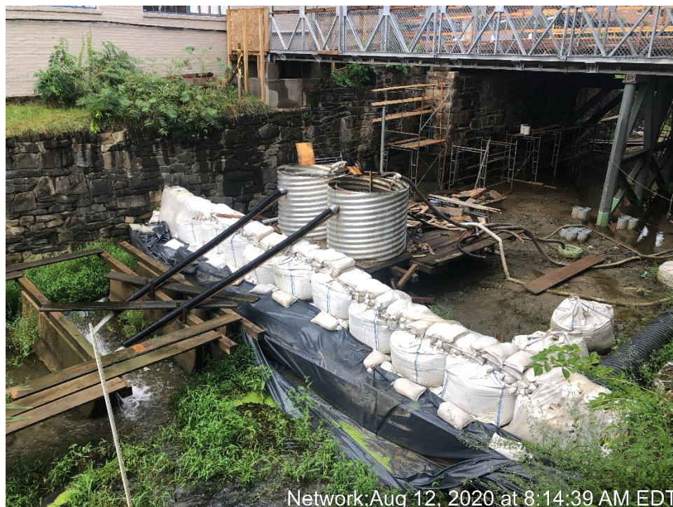
Dewatering the Work Zone
