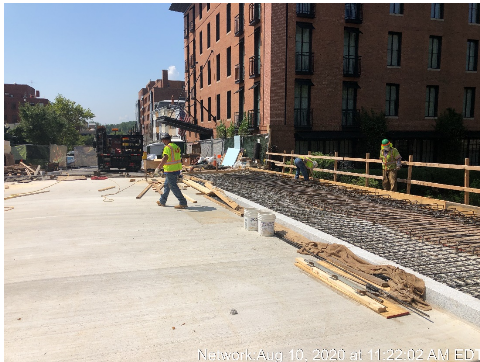
Placement of Reinforcing Steel for Sidewalk
