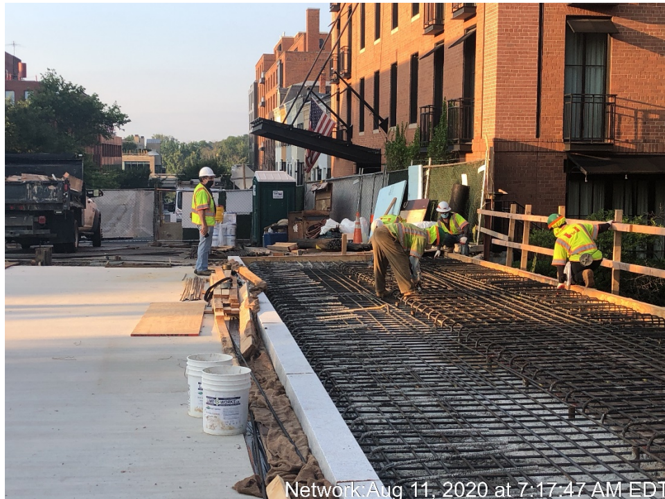
Placement of Reinforcing Steel for Sidewalk
