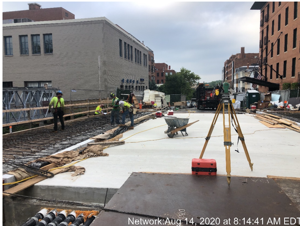
Placement of Reinforcing Steel for Sidewalk
