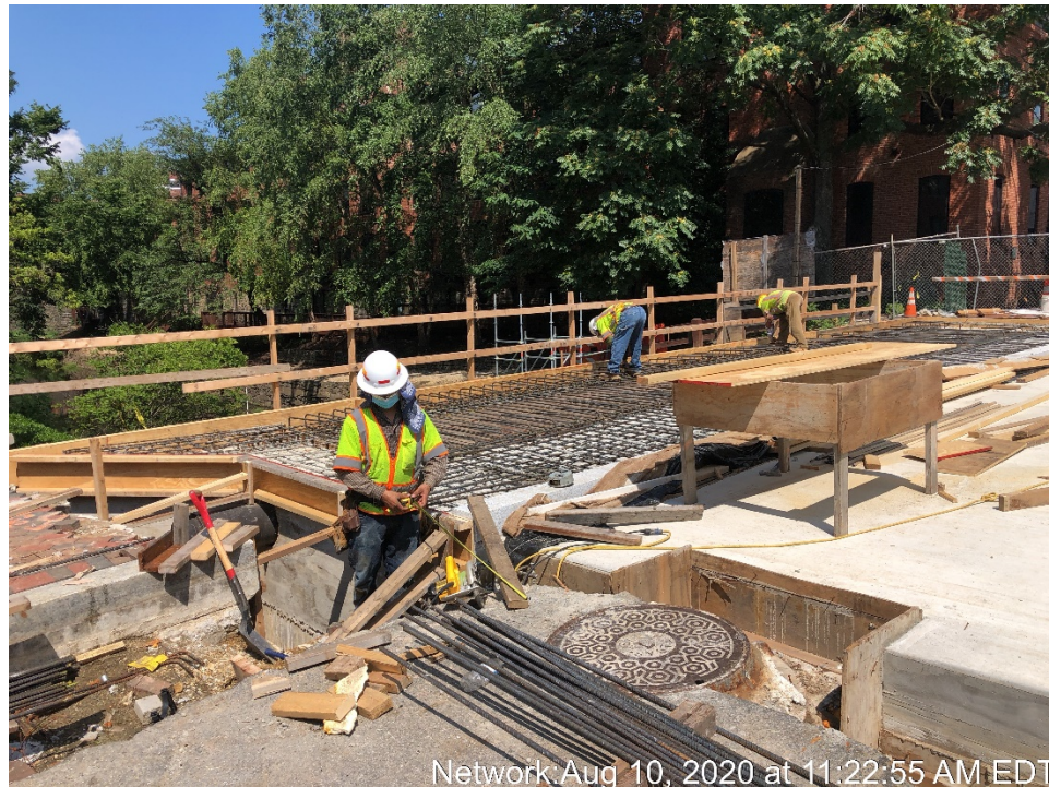
Placement of Reinforcing Steel for Sidewalk
