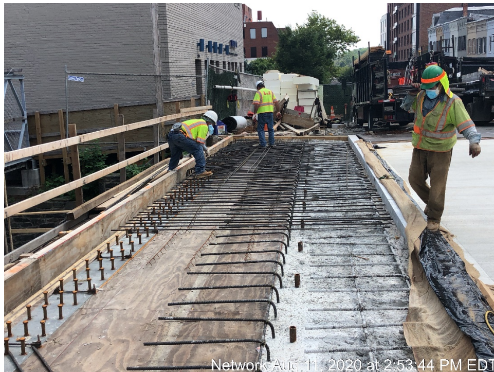
Placement of Reinforcing Steel for Sidewalk
