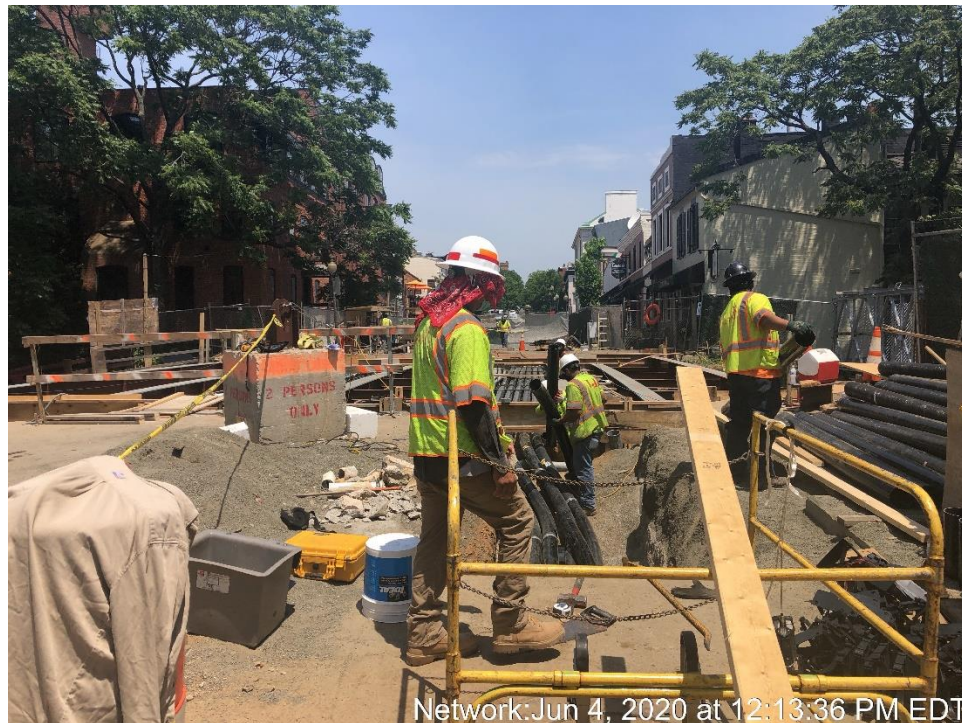
Installation of Pepco Conduits on North Side
