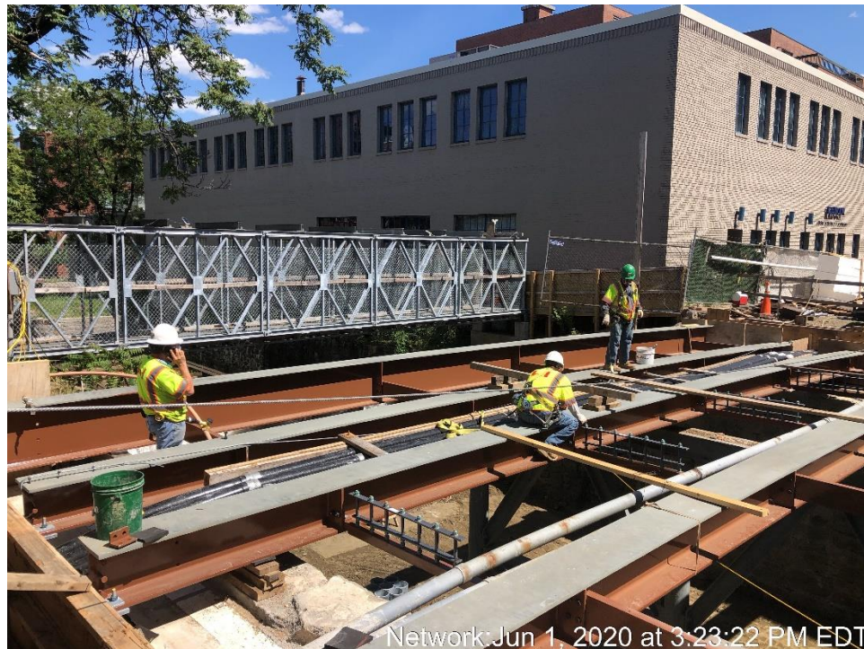
Installation of Utility Support
