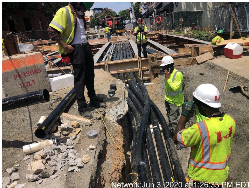
Network: Jun 3, 2020 at 8:42:20 AM EDT Installation of Utility Support
