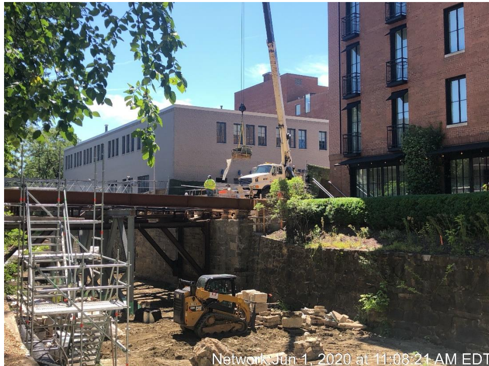
Removal of Rubble Stone from Canal
