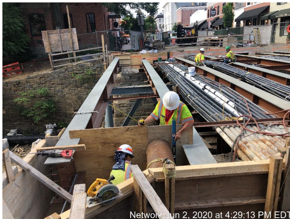
Network: Jun 2, 2020 at 11:58:38 AM EDT Installation of Utility Support
