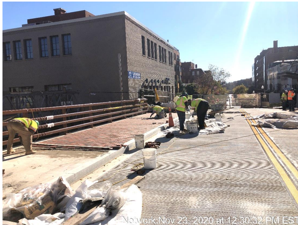
Construction of Brick Sidewalk – East Side of the Bridge
