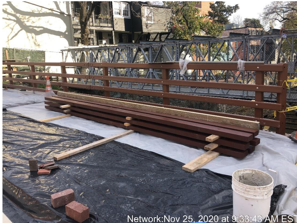
Painting of NPS Railing Posts
