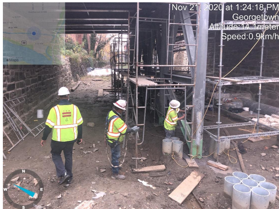
Epoxy Hole Filling at Pier Column
