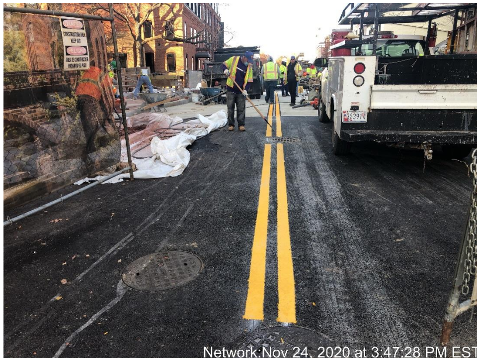
Thermoplastic Pavement Marking North Side of Bridge
