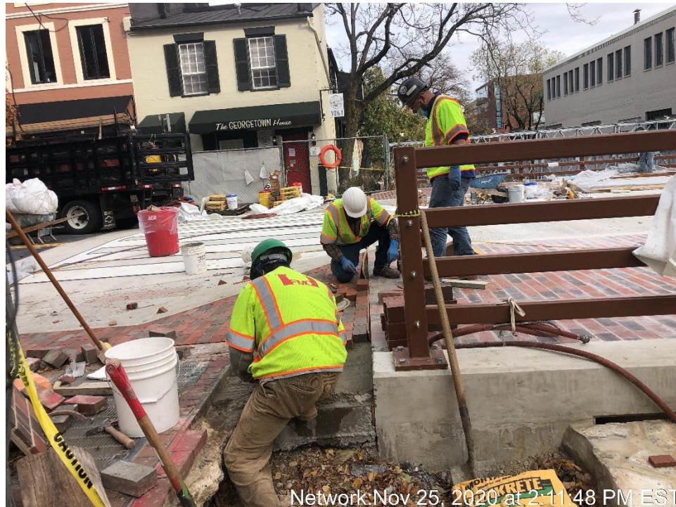
Construction of Brick Sidewalk – Northwest Corner of the Bridge
