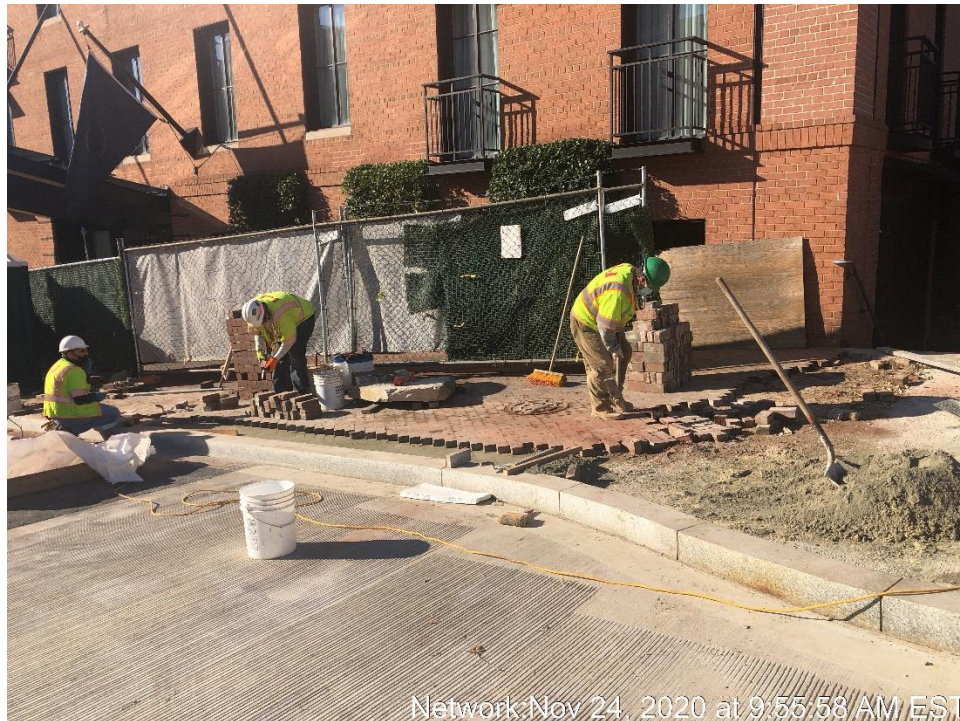
Construction of Brick Sidewalk – Southwest Corner of the Bridge
