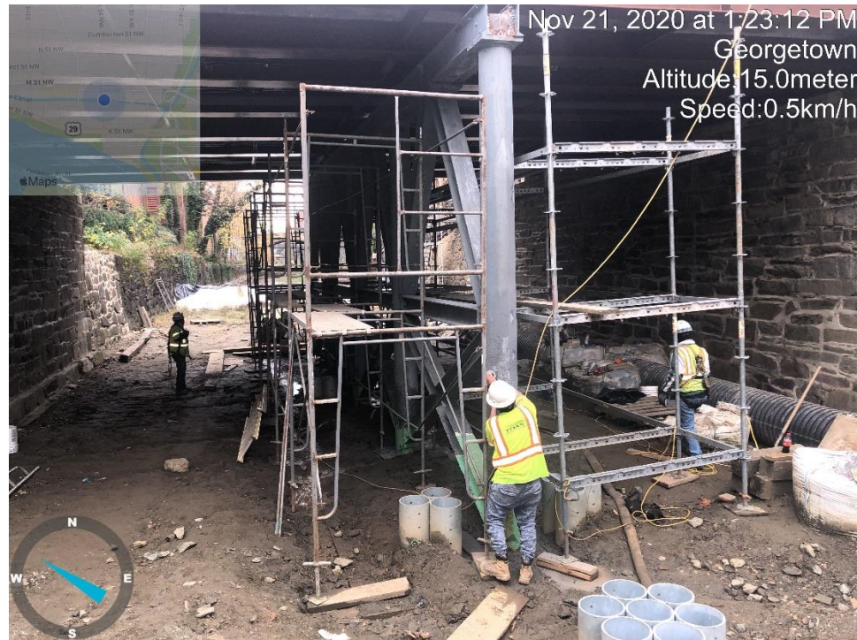
Epoxy Hole Filling at Pier Column
