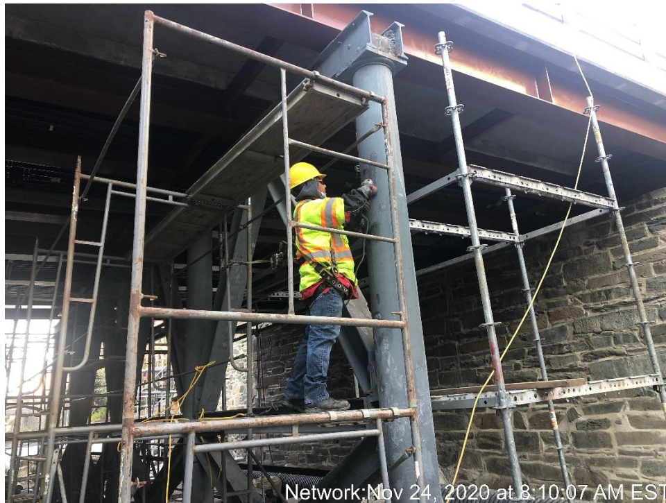
Epoxy Hole Filling at Pier Column
